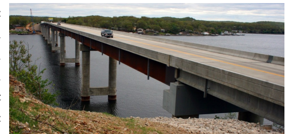
Fig 5: Photograph of New Hurricane Deck Bridge
