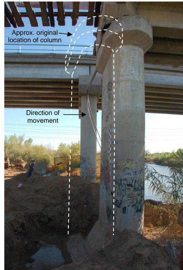
**Figure 2: Bent 5 of railroad bridge (foreground) that translated towards river causing unseating collapse, and Bent 5 of highway bridge (background) following 2010 El Mayor-Cucapah earthquake. Photo J. Gingery/GEER (2010).**
