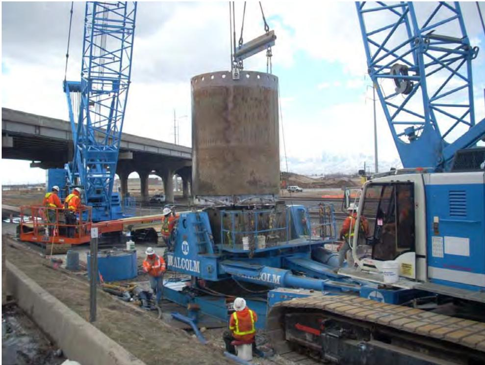
**Figure 1** Oscillator Constructing Drilled Shaft in Tight Quarters, I-15 Beck St. Crossing
