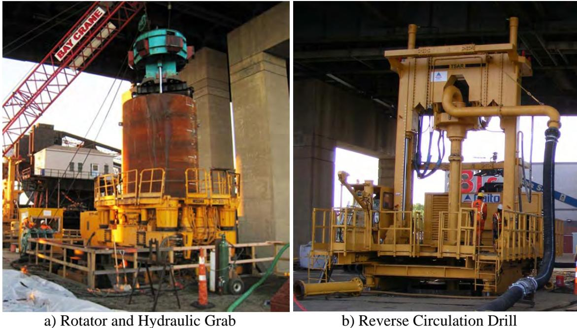
**Figure 7** Construction Equipment Working in Limited Overhead Clearance
