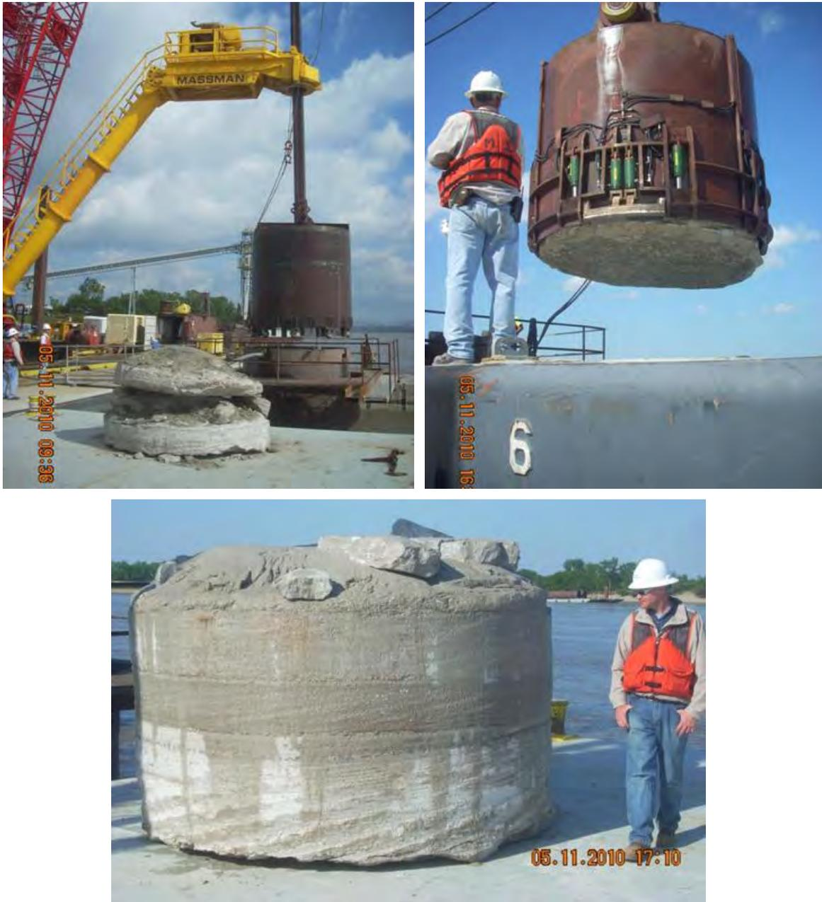
**Figure 5** Limestone Rock Extracted During Construction of Load Test Shaft
