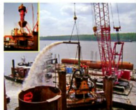
Shaft excavation using oscillator
