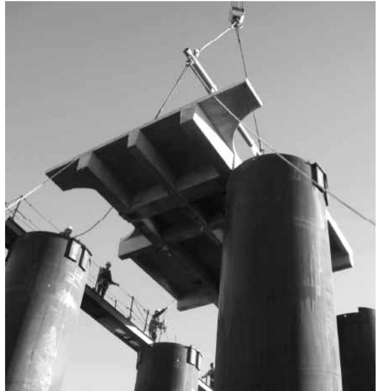
Figure 3. East Pier, Soffit Panels Erected.
