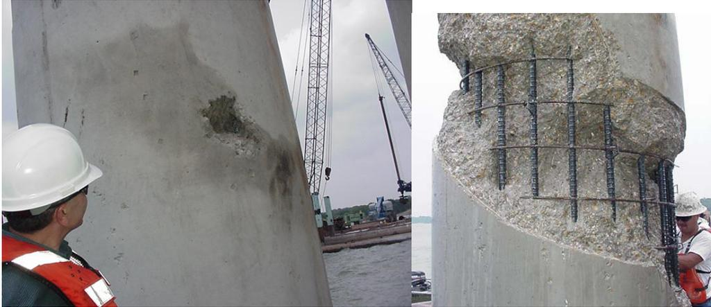
Figure 1 Surface flaws in concrete (left), after removal for repair (right)
