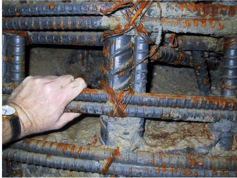
Figure 3 Defect in Shaft with Double Rebar Cages
