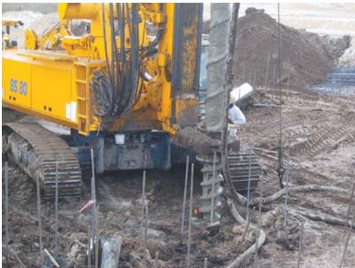
**Figure 3 Partial or Intermediate Displacement Pile Rig**
