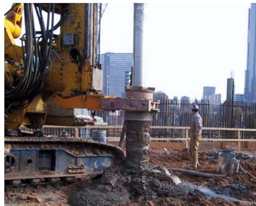
**Figure 4 Full Displacement Pile Rig**
