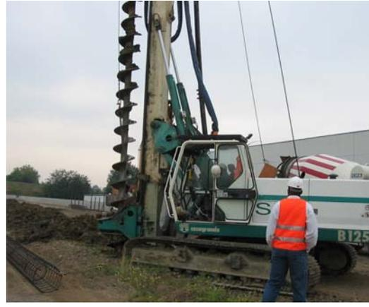
**Figure 2 Hydraulic CFA Rig**
