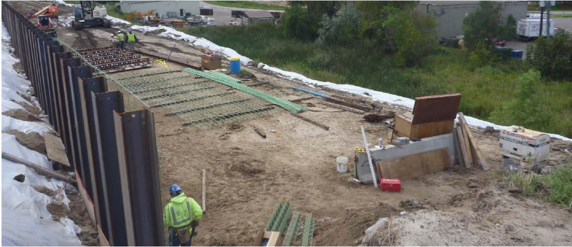
Figure 9. HP 18 x 135 piles were driven to provide stability to the roadway.
