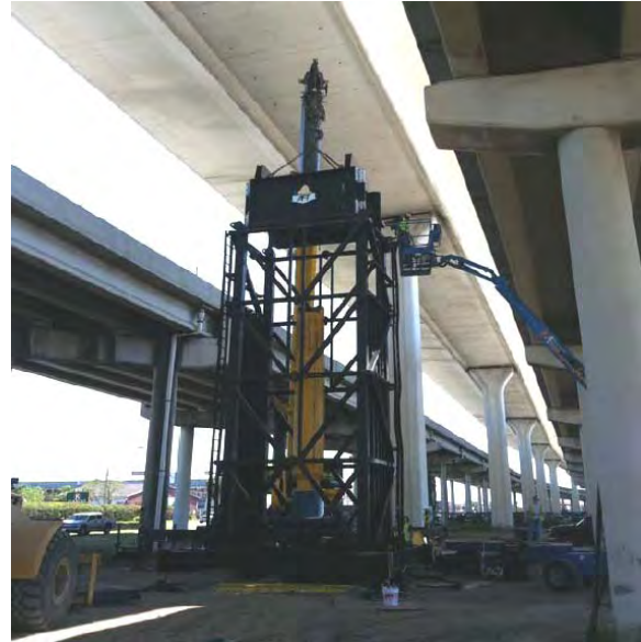
Figure 7. Statnamic Testing, Selmon Widening Project.
