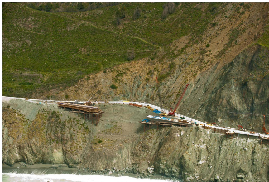
Figure 4. Trestles extending from north and south abutments.
