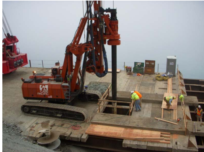
Figure 5. Drilled shaft excavation from south trestle.
