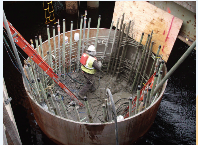
GILMERTON BRIDGE - Chesapeake, Virginia
