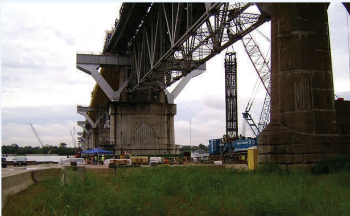
HUEY P. LONG BRIDGE WIDENING - New Orleans, Louisiana
