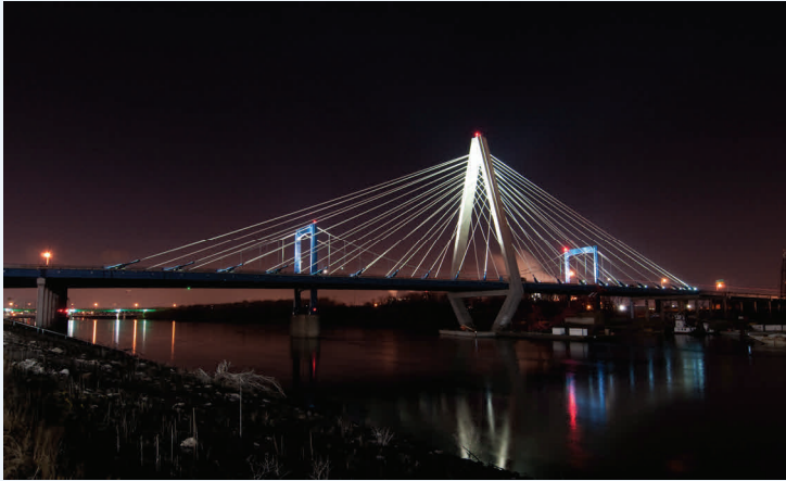
CHRISTOPHER S. BOND BRIDGE - Kansas City, Missouri
