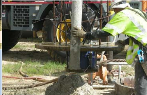
16in O-cell with 20in base plate (Test Shaft 2)
