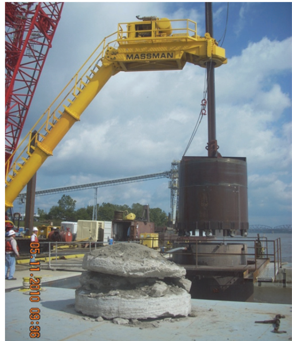
Figure 4 Coring at the Load Test Shaft
