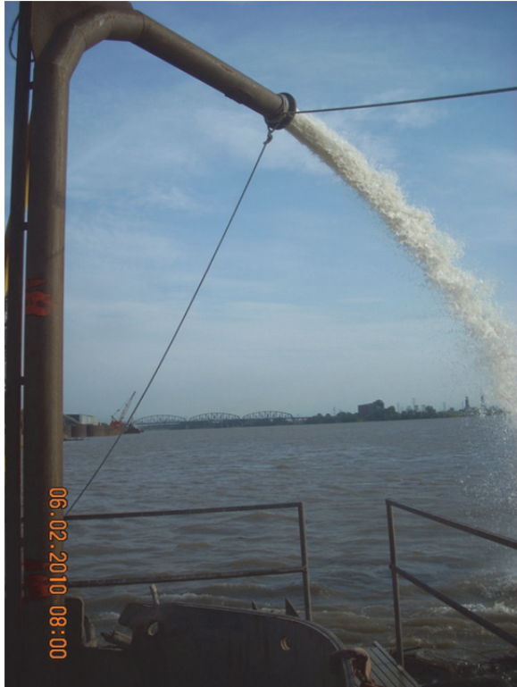
Figure 6 Air Lifting the Shaft Excavation
