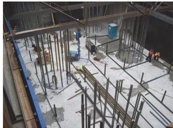
Figure 8 Cofferdam at East Pier
