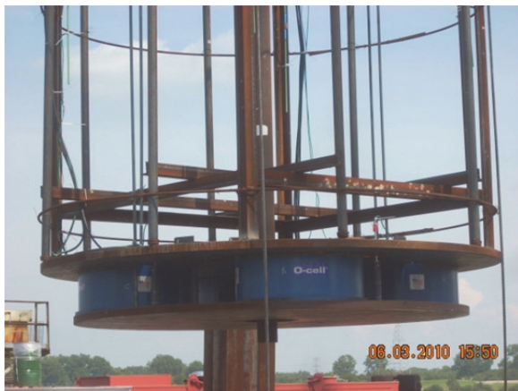
Figure 7 O-cell Assembly
