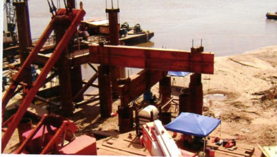
Load test setup
