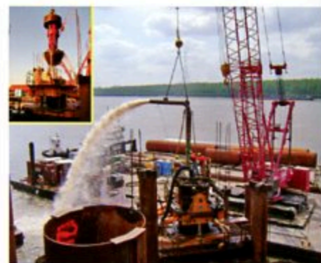
Shaft excavation using oscillator
