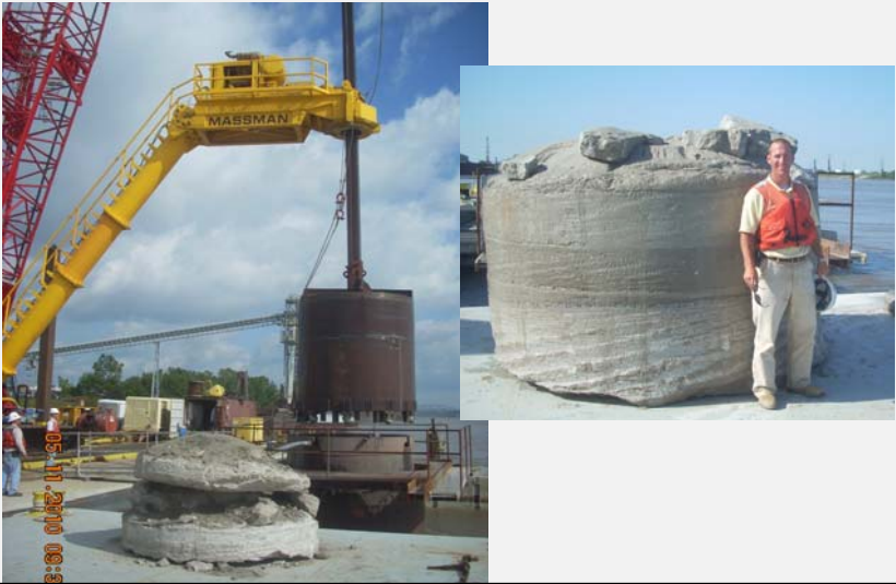
Construction of Load Test Shaft
