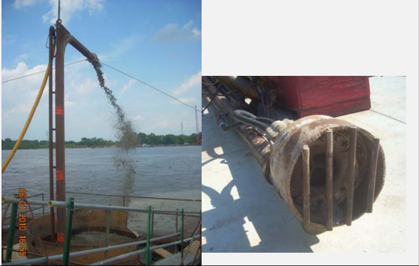
Construction of Load Test Shaft
