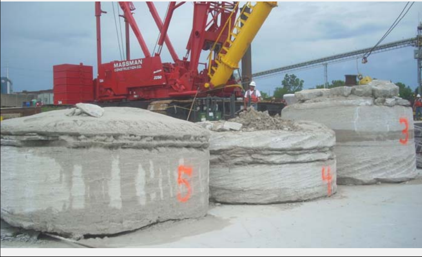
Construction of Load Test Shaft
