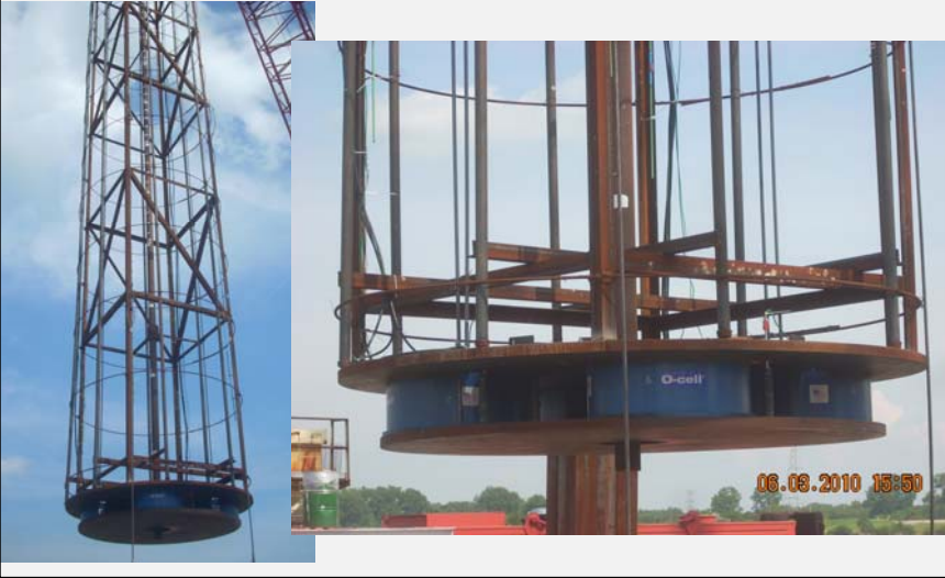
Construction of Load Test Shaft
