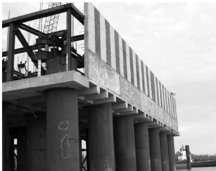
Figure 4. East Pier, Structural Bracing and Precast Walls Installed
