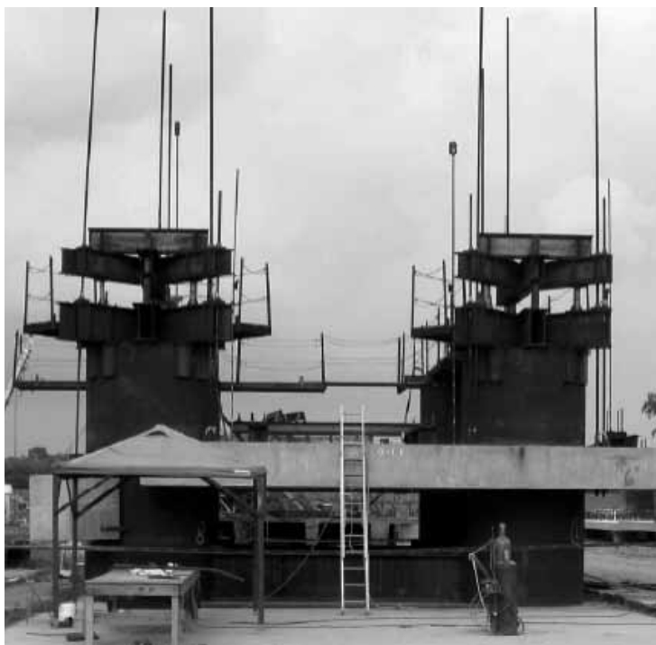
Figure 11. Lowering Training Mock-Up
