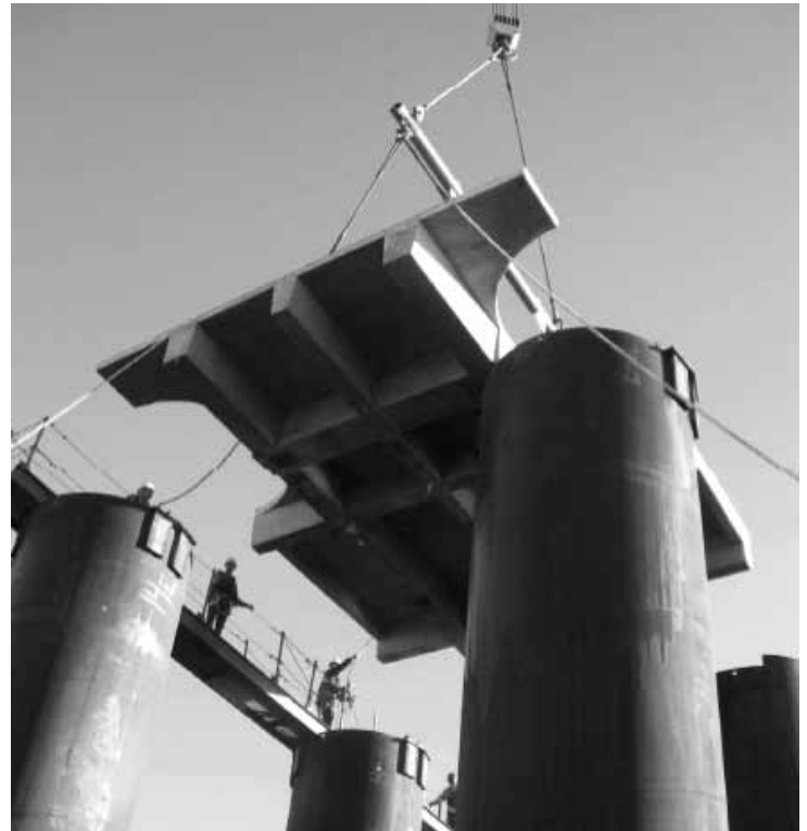
Figure 3. East Pier, Soffit Panels Erected.
