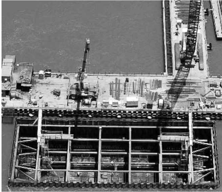
East Cofferdam Upon Completion of Lowering 47 feet
