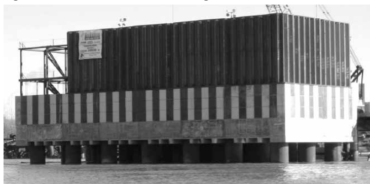
Figure 5. East Pier, Upper Structural Bracing and Sheet Pile Follower Installed
