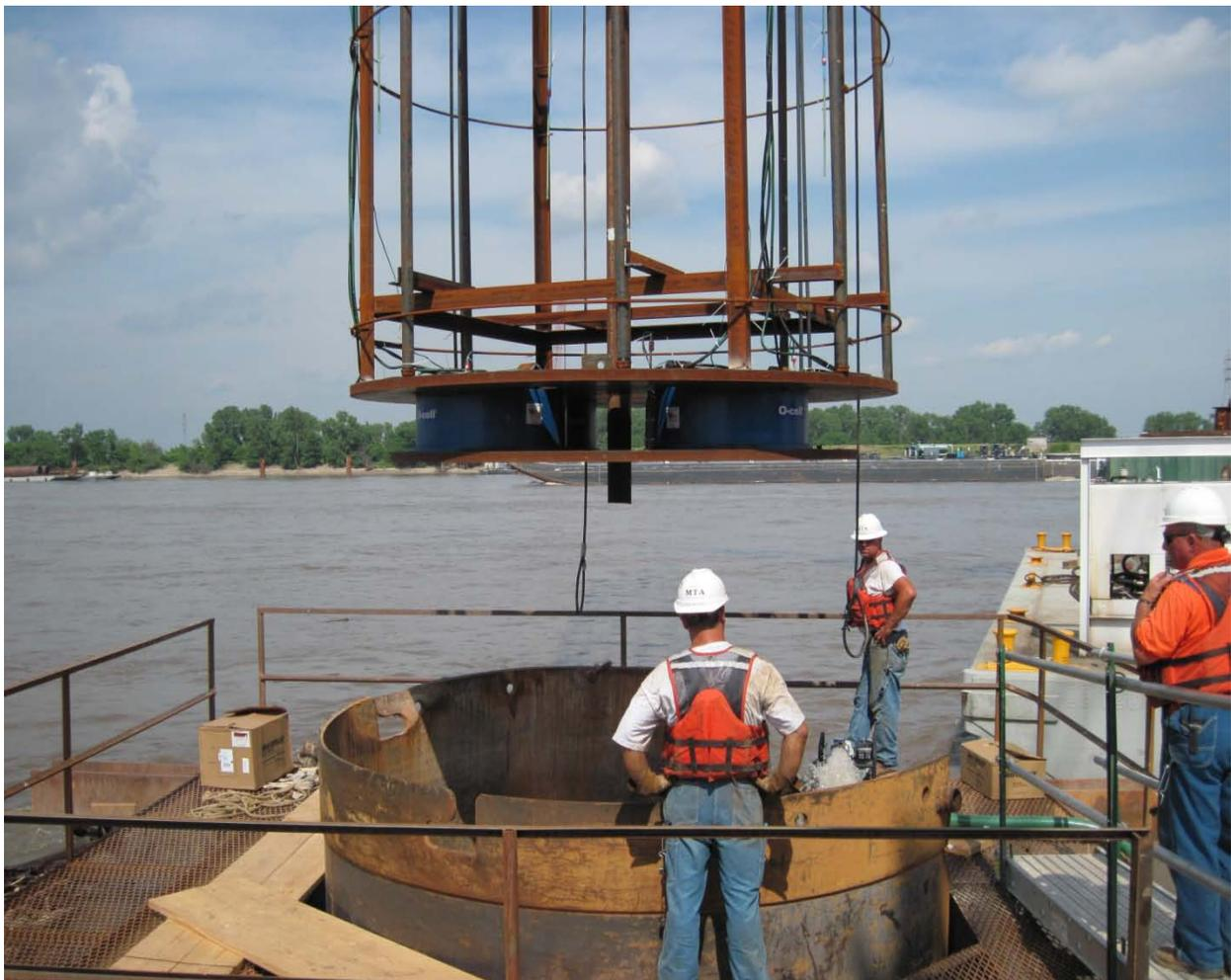
MTA workers prepare to lower the load testing system into a shaft drilled into rock beneath the Mississippi River.
