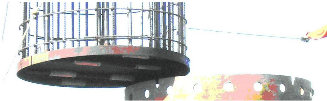
**Figure 3. Sleeve-Port with Top Plate Grouting Mechanism.**
