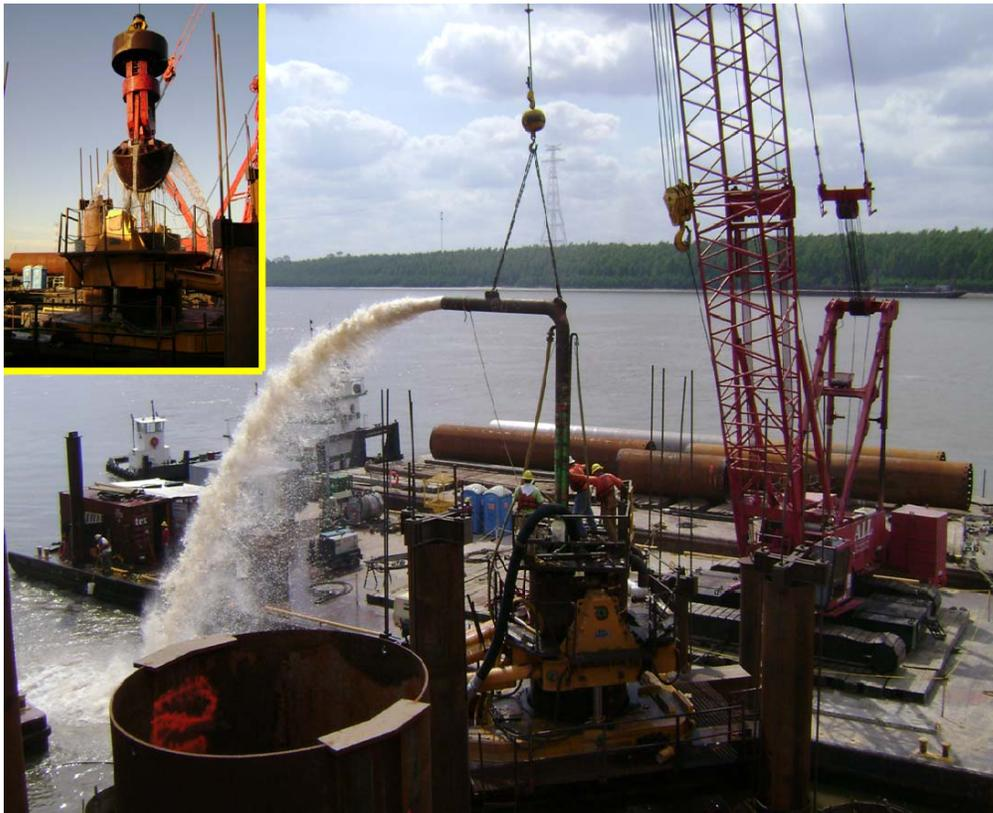
**Figure 2. Shaft Excavation Using Oscillator, Grabs, and Air-lift.**
