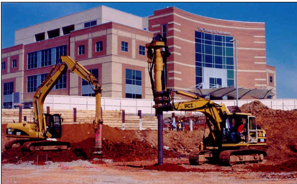
Figure 6. Geopier Construction at Project Site
