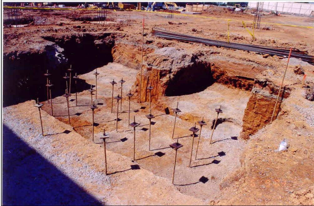
Figure 5. Uplift Anchor Rods in Subgrade
