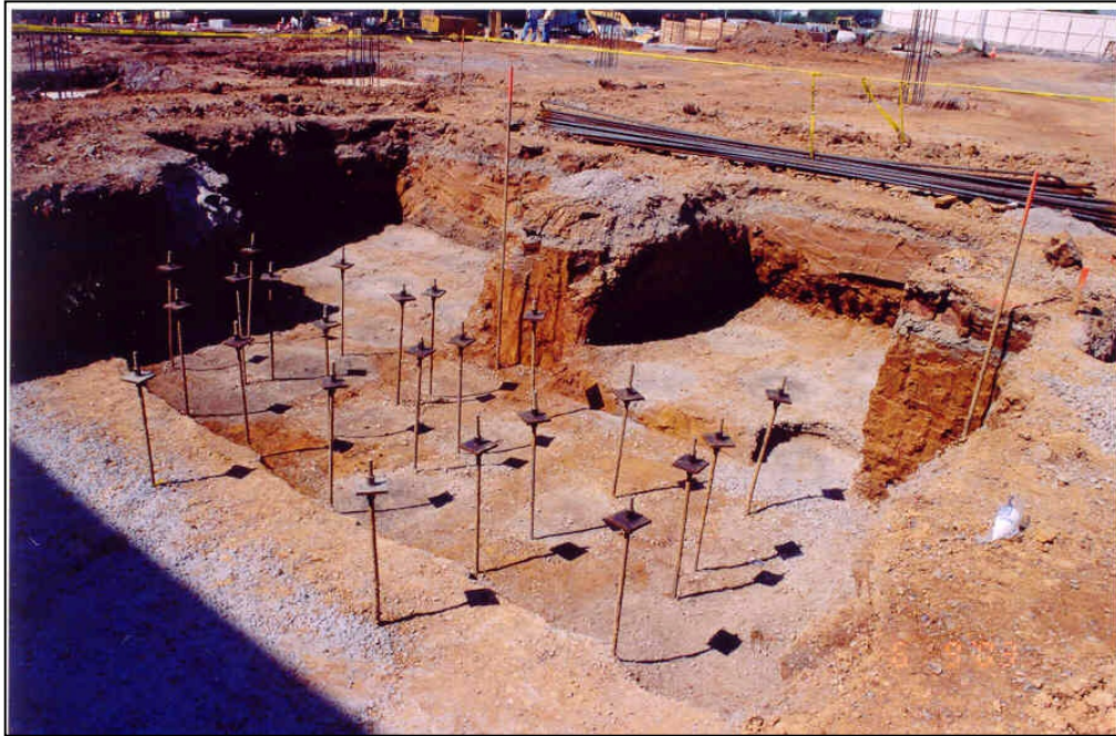
Figure 5. Uplift Anchor Rods in Subgrade
