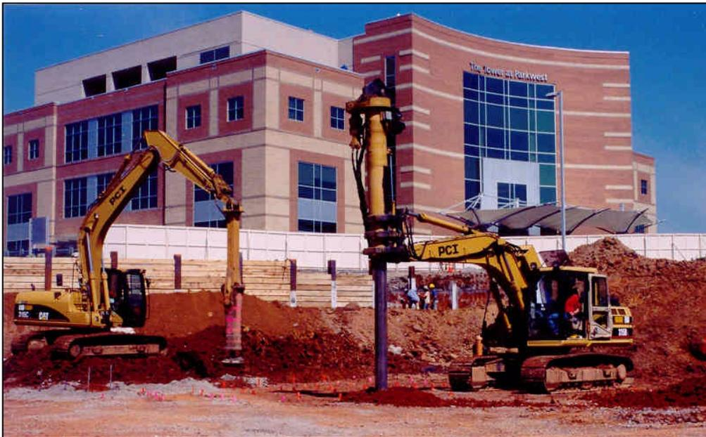
Figure 6. Geopier Construction at Project Site
