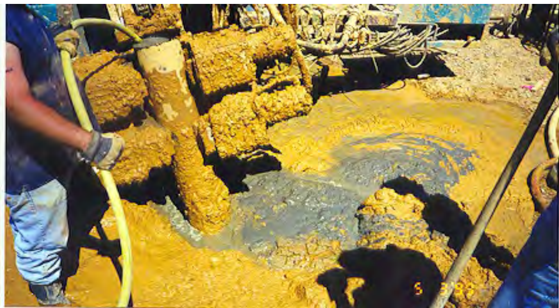
Figure 2. Disturbed Soil after Micropile Installation
