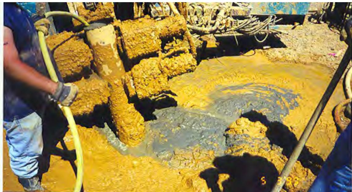
**Figure 2. Disturbed Soil after Micropile Installation**
