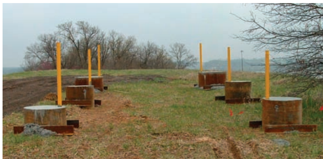
[FIG. 2a] Test Shafts
