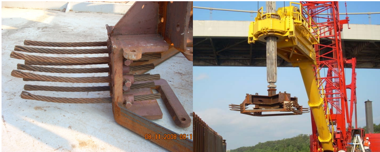
Figure 9: "Back-scratcher" for Preparation of Rock-Socket Sidewall
