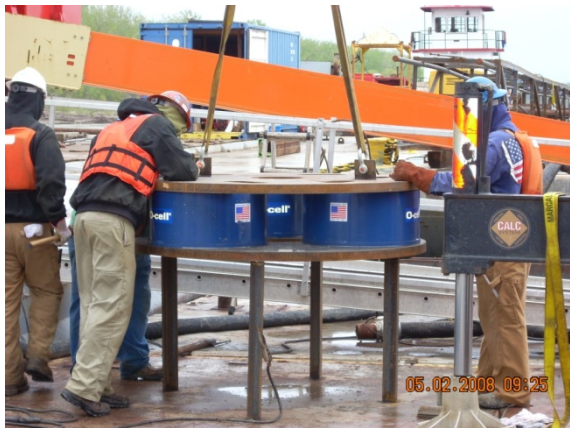
Figure 11: Three O-cells attached top and bottom to 2-in thick steel plates.
