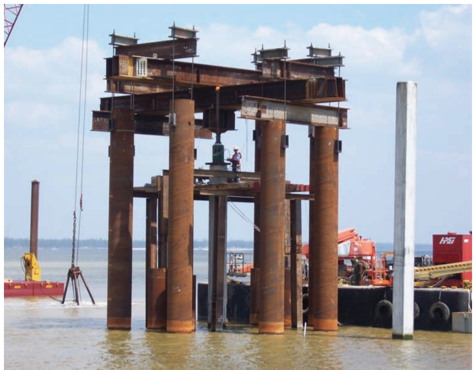
[FIG. 2] Conventional Static Load Test
