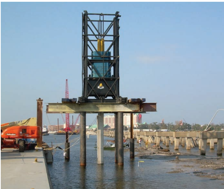
[FIG. 3] Statnamic Load Test
