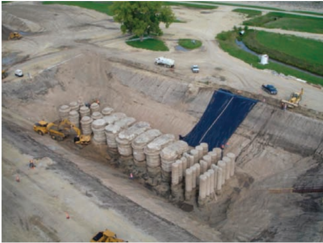
[FIG. 1] (b) Jet grout and soil mix columns during excavation
