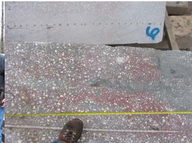
Figure 11 SCC Mix, View of Mixing in Upper 13 ft.
