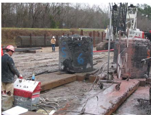
Figure 6 Wire Saw Operation
