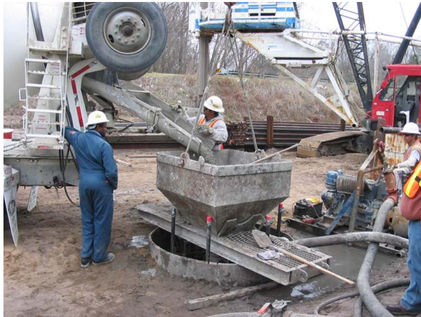
Figure 2 Tremie Placement of Concrete
