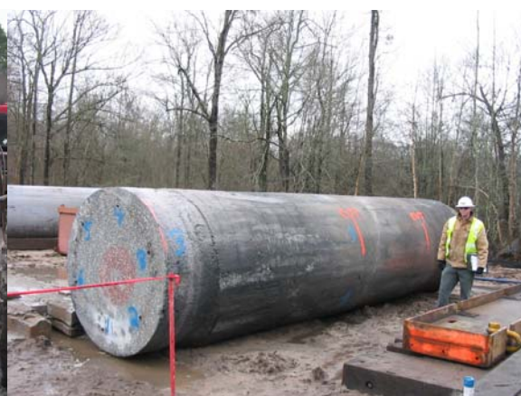
Figure 7 SCC Shaft after First Cut
