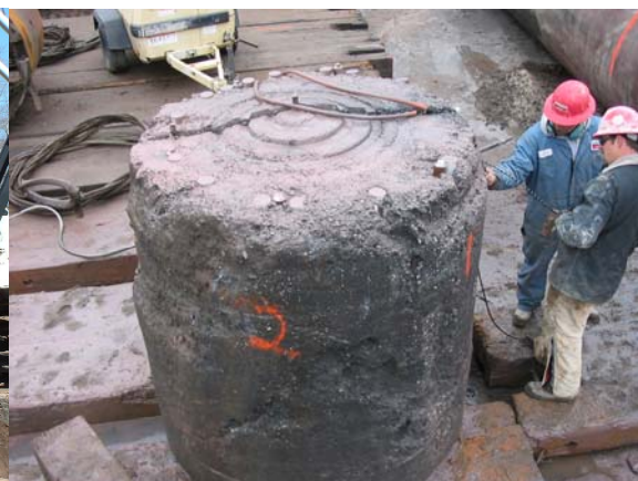
Figure 5 Shaft Base (Bottom 6 feet)
