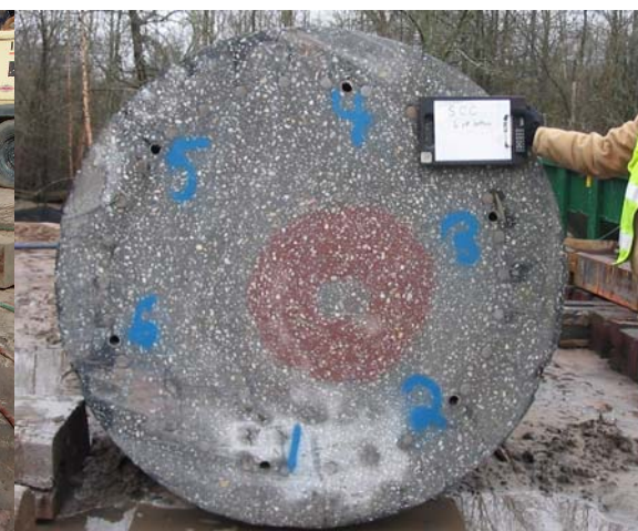
Figure 9 Section of SCC Mix, 6 ft from Base
