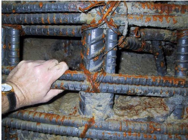
Figure 3 Defect in Shaft with Double Rebar Cages and 1 inch Maximum Aggregate
