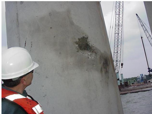
Figure 2 Trapped Laitance in a Shaft Observed after Casing Removed
