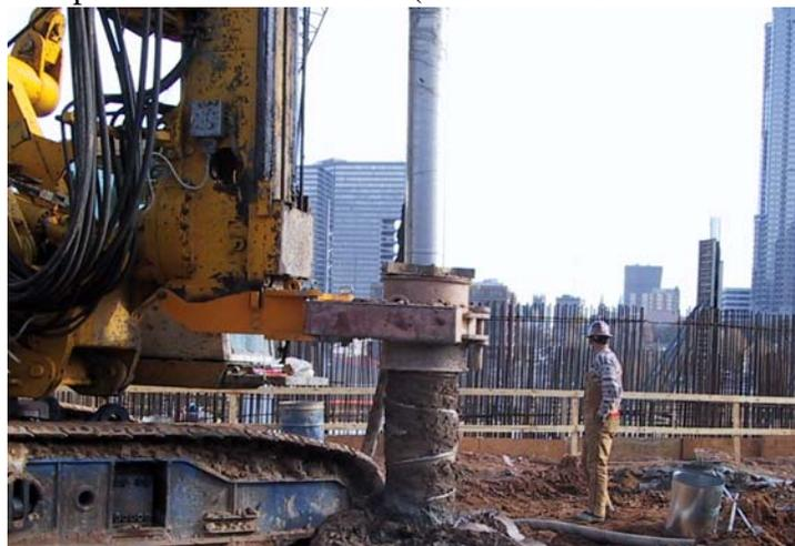
**Figure 8 Drilled Displacement Pile Installation**
