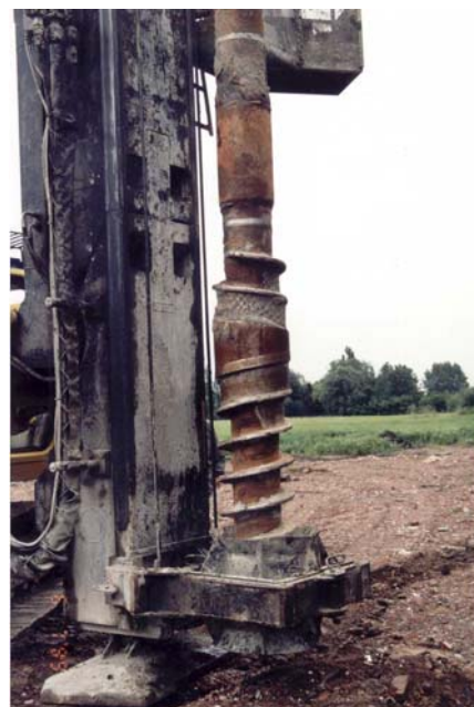
Figure 3 Intermediate (Partial) and Full Drilled Displacement Piles
