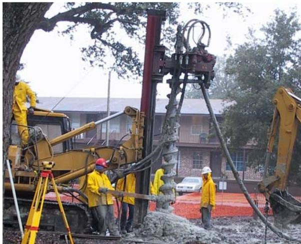
**Figure 5 Low Headroom CFA Pile Application**
