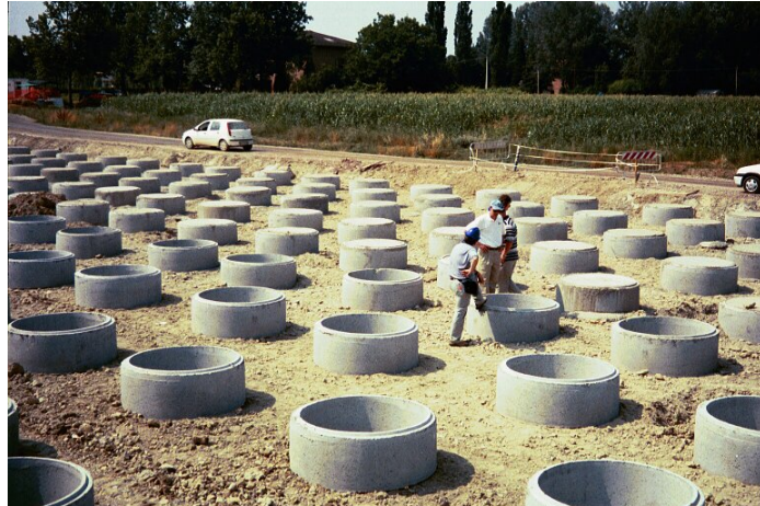
Figure 4 Railway Embankment to be Supported on CFA Piles
