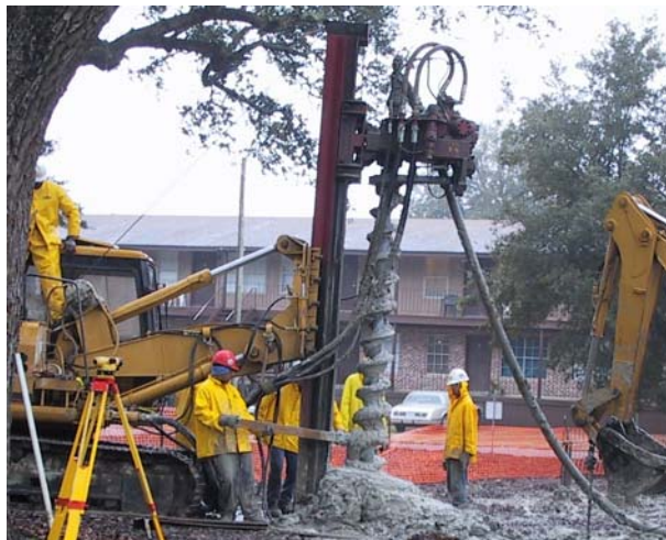
Figure 5 Low Headroom CFA Pile Application
