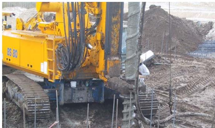
**Figure 3 Intermediate (Partial) and Full Drilled Displacement Piles**
