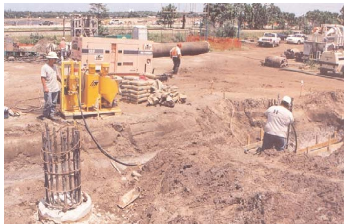
Post Grouting of Production Shafts
