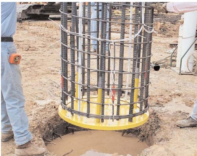
Grout Distribution System on Shaft Base
