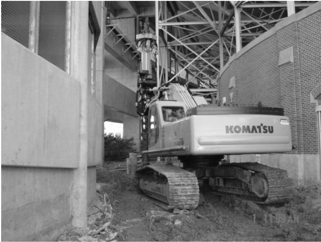
Figure 2 – Lo-Drill operating in confined work area.
