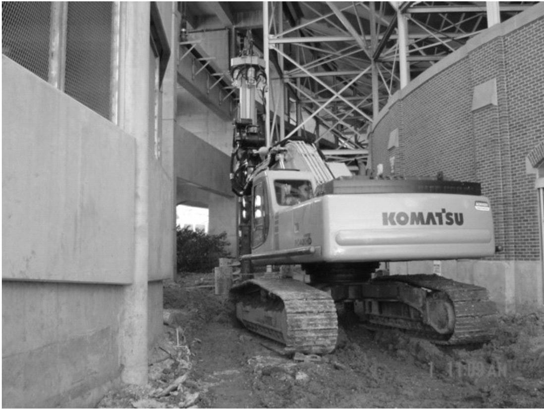
**Figure 2** – Lo-Drill operating in confined work area.
