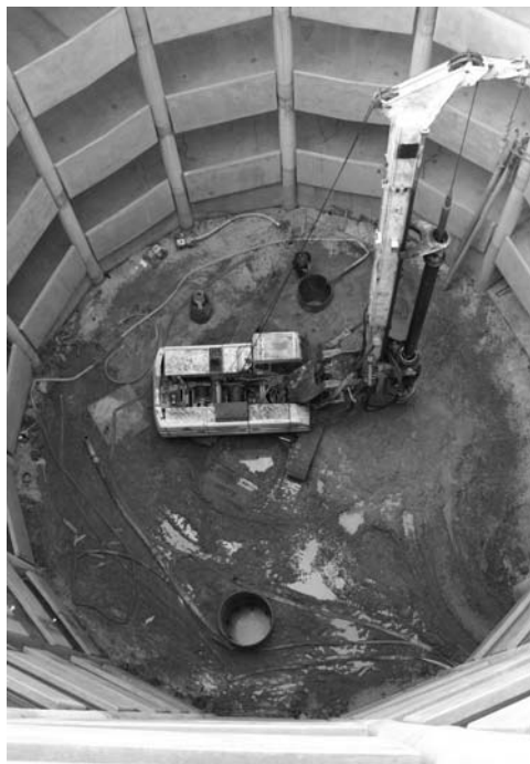
Figure 3 – Installing Drilled Shaft in Upper Deck Ramp Structure.
