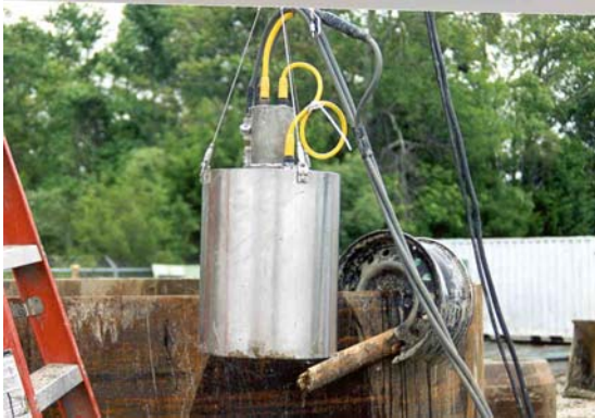
Figure 2 Mini SID Device for Inspection Of Shaft Base Conditions
